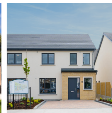
Ravens Mill Rolestown, Co. Dublin
