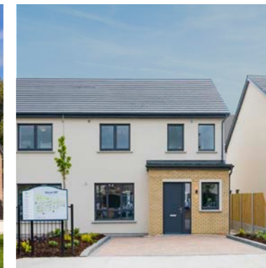
Ravens Mill Rolestown, Co. Dublin
