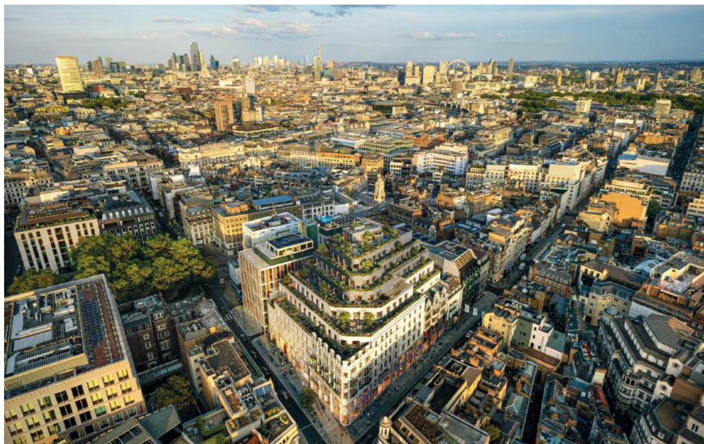
Renewed purpose Office and retail at 7 Brook St in London's Mayfair
