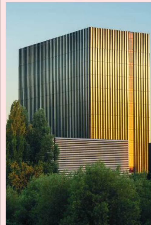
Number crunching Data centres use huge amounts of power
